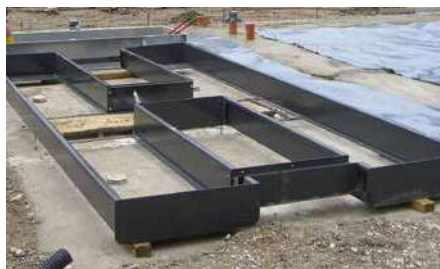
Mounting frame for runway versions with or without floor compensation for accurate lift fitting. The prefabricated edging frames ensure high accuracy during installation.
